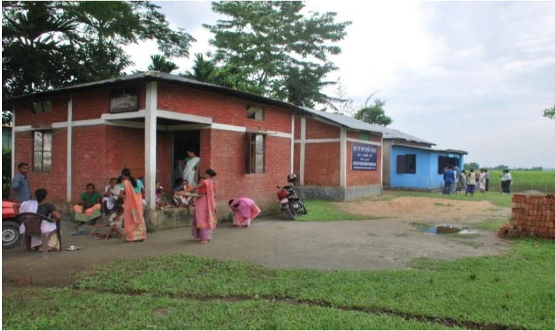
The school and the Anganwadi Centre complex
